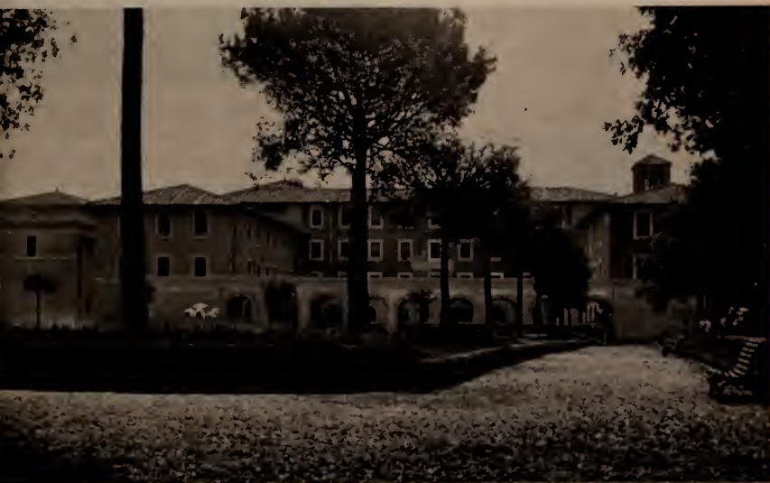
View of new Curial wing at SS. Giovanni e Paolo Monastery. The aula where the General Chapter was held is located in this wing, center. Library (older) at far left.
