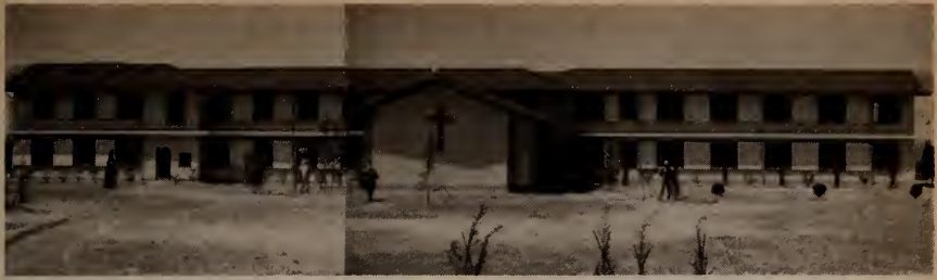
Retreat House From Chapel Side
